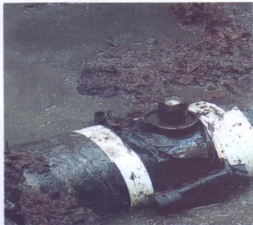
Fig B: picture taken after excavation.
