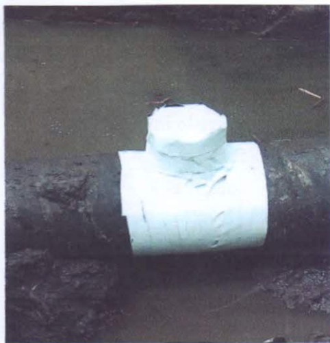
Fig C: picture taken after wrapped.
