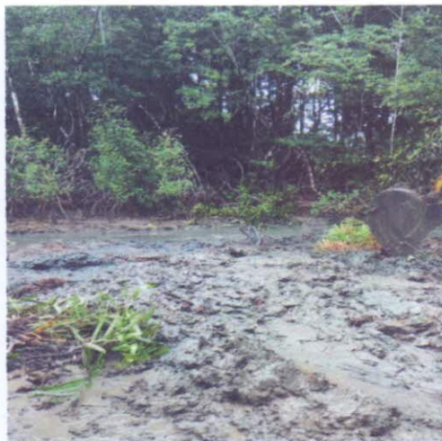
Fig D: picture taken after backfilled.
